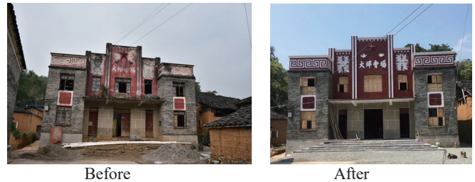
Fig. 2 Before and After the renovation of the daping Conference place
